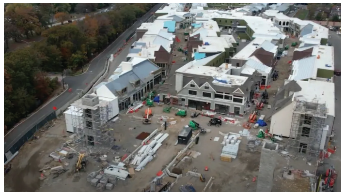
Belmont Park Village under construction.
