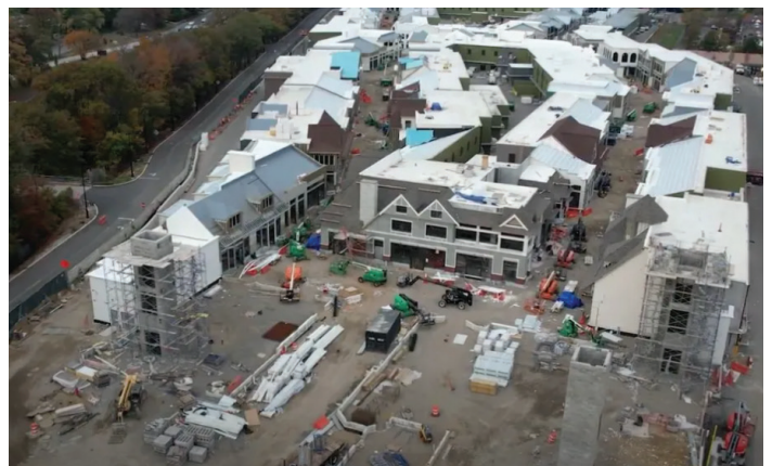
Belmont Park Village under construction.
